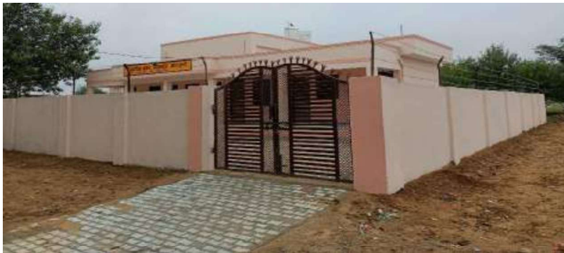
Construction of Community Centre at New Mohanpura Village
