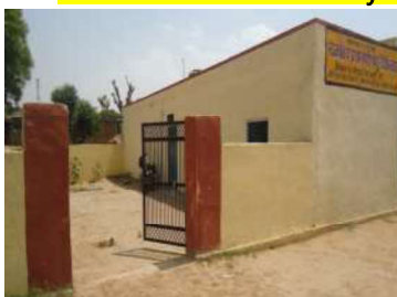
Renovation of Veterinary Hospital at Gordhanpura
