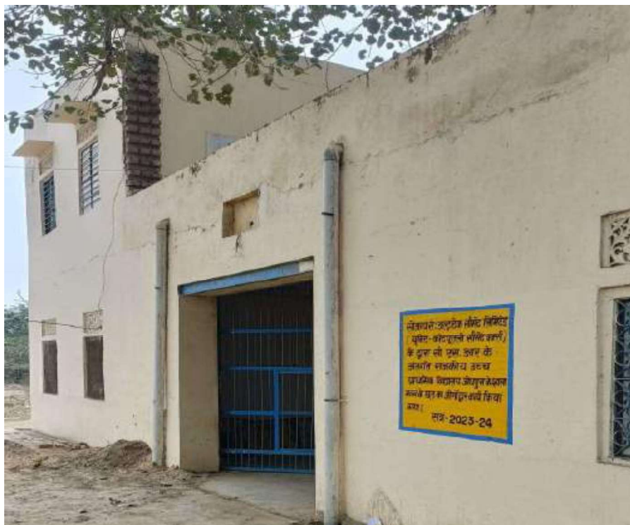
Jodhpura school building roof top work
