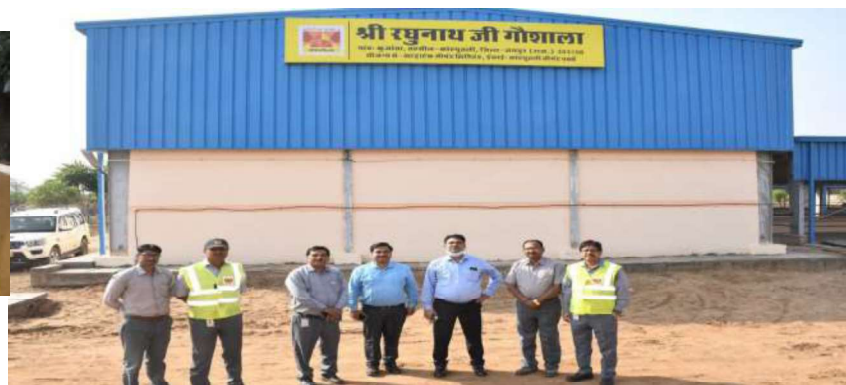
Construction of Gaushala near Kujota Village
