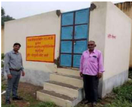
Construction of Toilet in Govt. School Kujota
