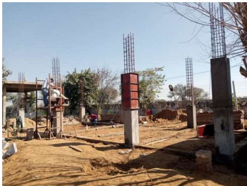
Store Room Construction at Gaushala
