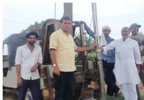
Construction of Borewell at Mohanpura
