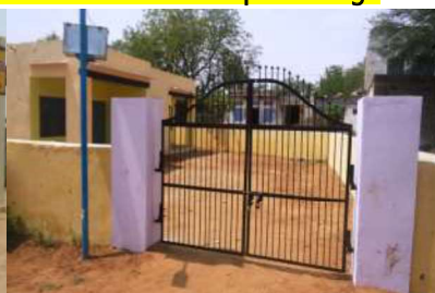
Renovation of Health Sub Centre at Gordhanpura
